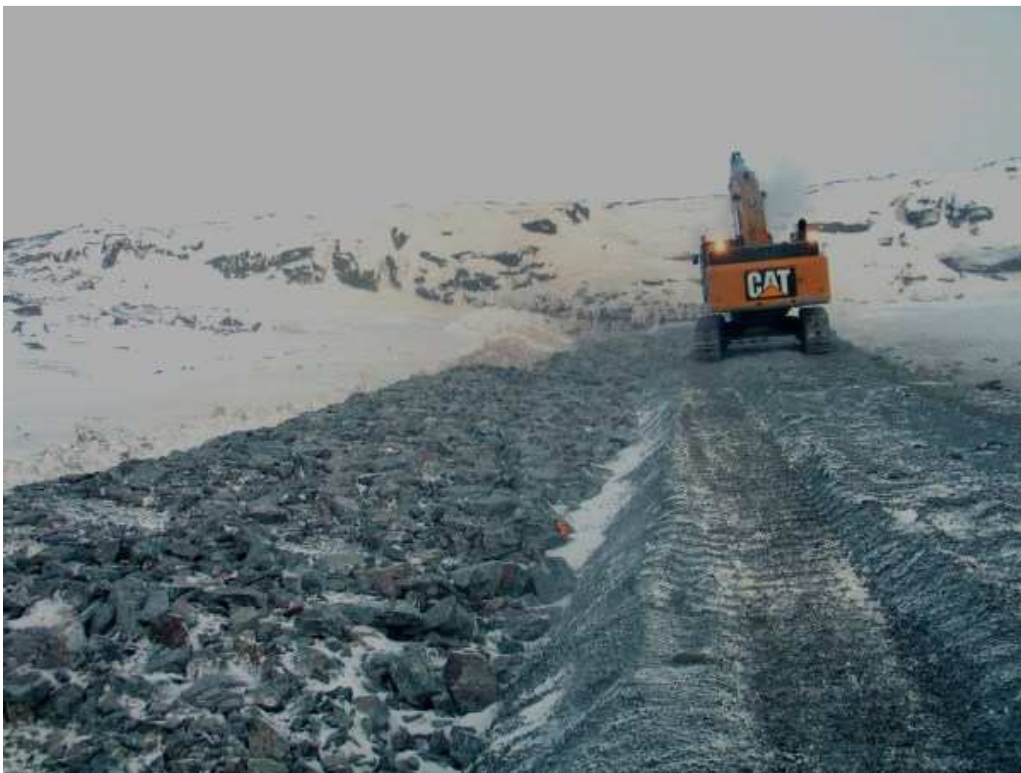
Photo 9: Progress filling key trench.
