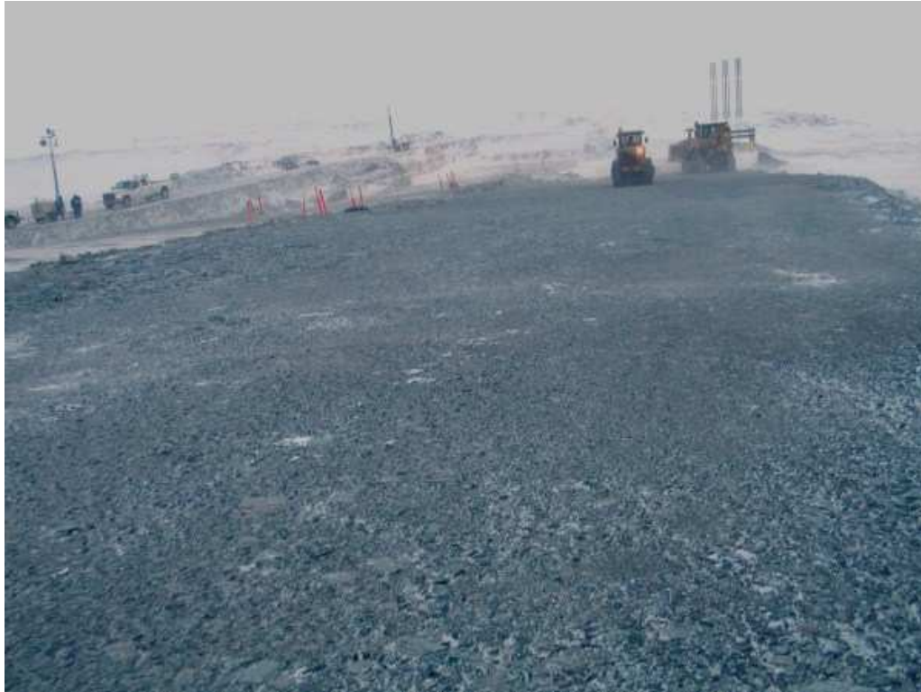
Photo 8: Dam shell construction. Vibratory packer worked most of the day.
