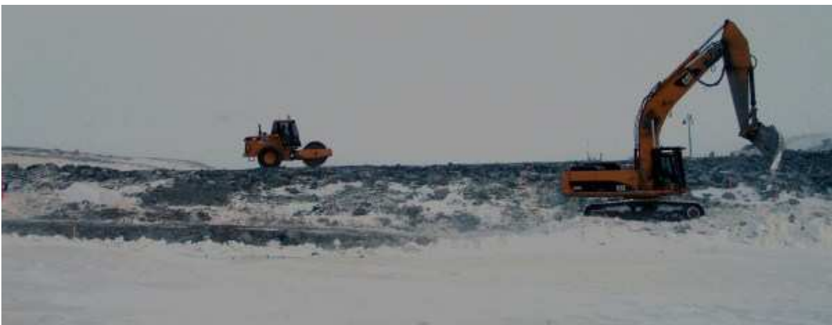
Photo 7: Excavator sloping down stream ROQ
